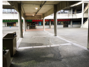
3 Basketball Courtyard Table - Near Library
